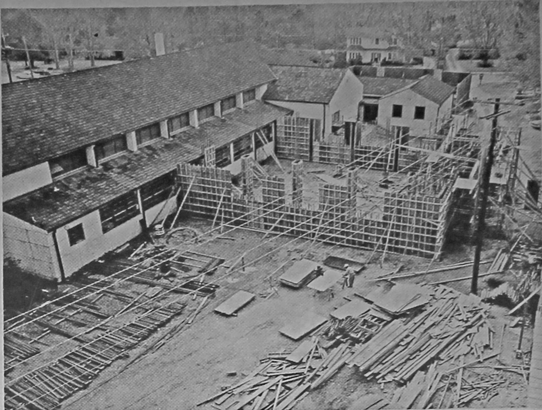
Enlargement of the cafeteria is well underway. Workmen erect forms for the concrete exterior walls on the north side of the existing building. Construction in foreground is added dining area, and walls at right rear of the building will be part of addition to enlarged kitchen and storage area. The exterior additions will be blended into the existing structure to make for a pleasing appearance.
